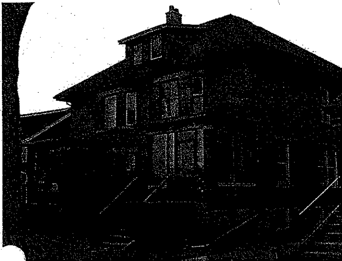
chimney with two pots, and shaped-block foundation.
